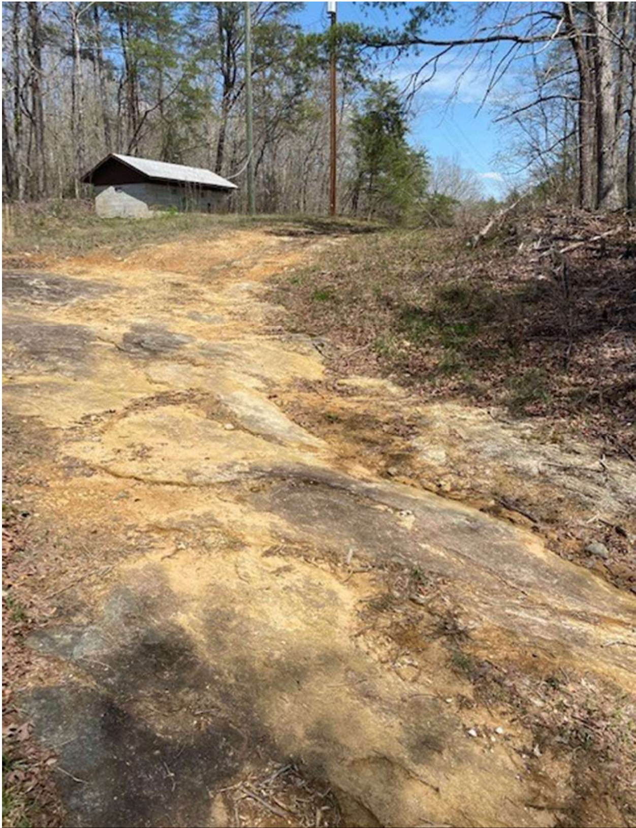
This is a photo of the building on top of the hill that houses the 24" check valve. This is also the site for the future building that will house the new VFD's.
